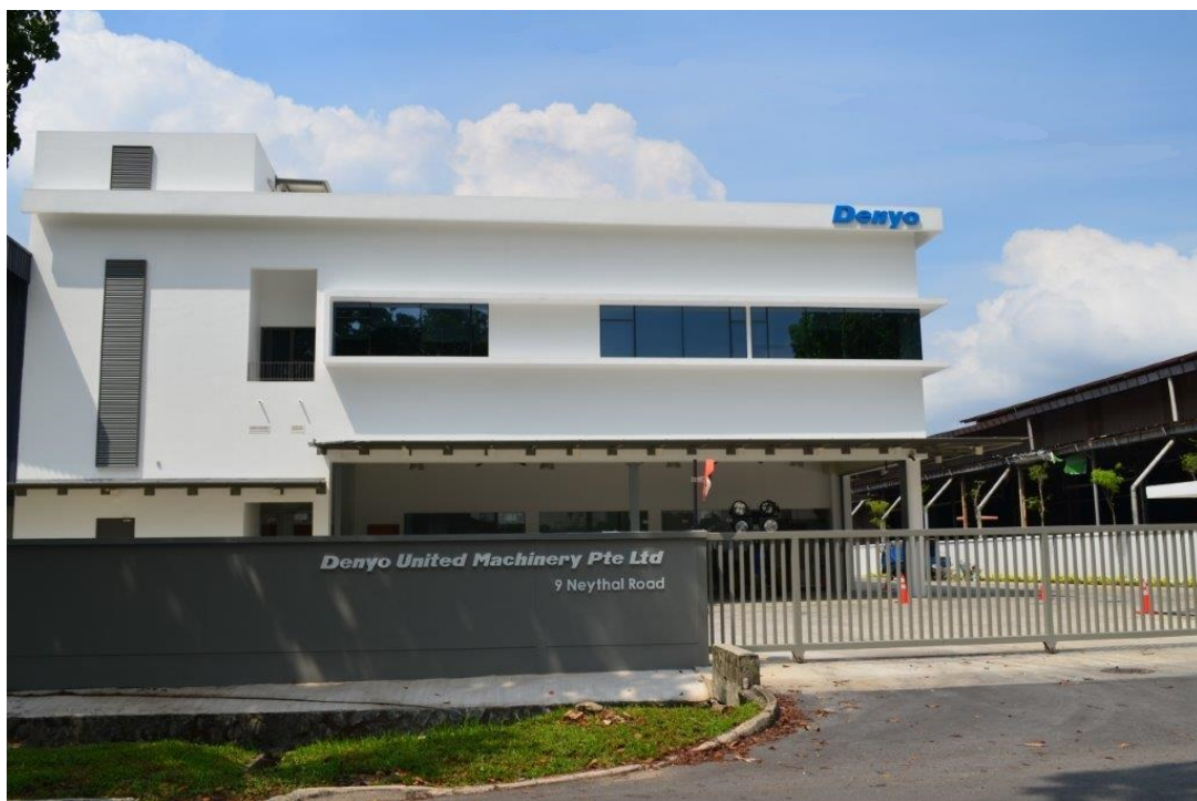
写真 : Denyo United Machinery Pte Ltd (Singapore)
