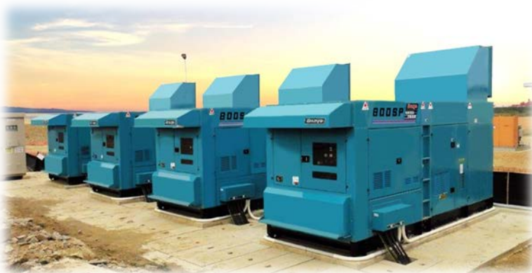
Generators installed on a plant construction site overseas
