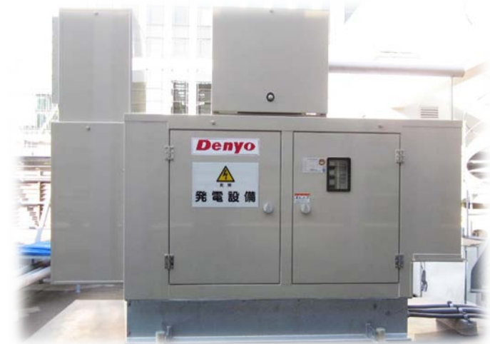
Backup generator installed at financial institution
