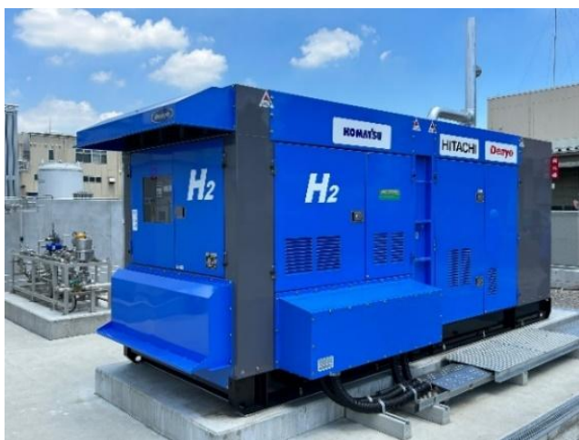
Hydrogen-light oil mixed combustion Generator delivered Komatsu Oyama Plant
