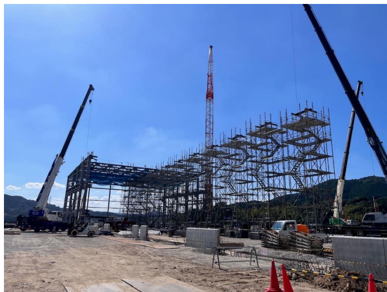
New plant under construction (NISHIHATSU, Karatsu City, Saga Prefecture)
