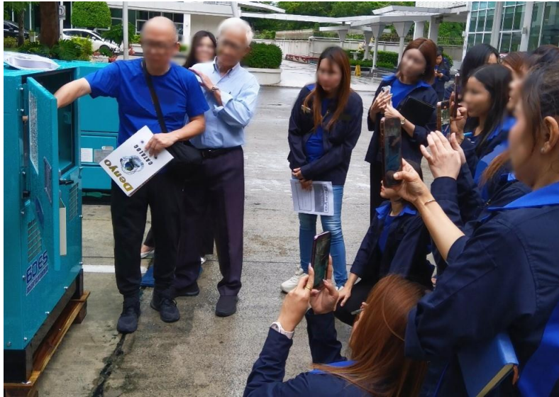
Operation of an installed power generator(Thailand)
