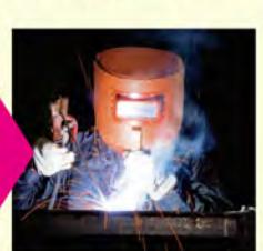
Resume welding works.
