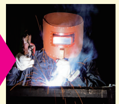
Resume welding works.
