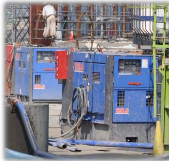
Construction work in the Tokyo Metropolitan Area
