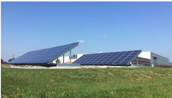
30 kW solar panels
